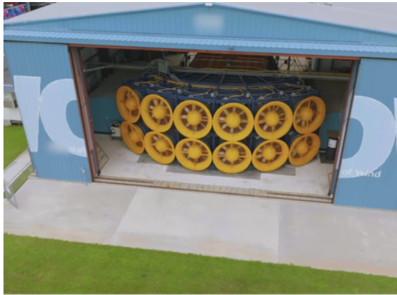
WIND TESTING FACILITY
