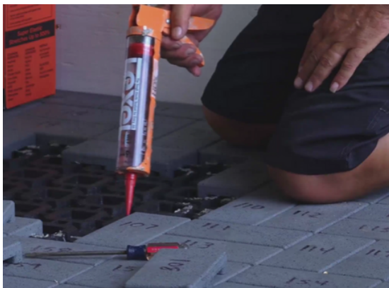
ADHERING PAVERS WITH ADHESIVE
