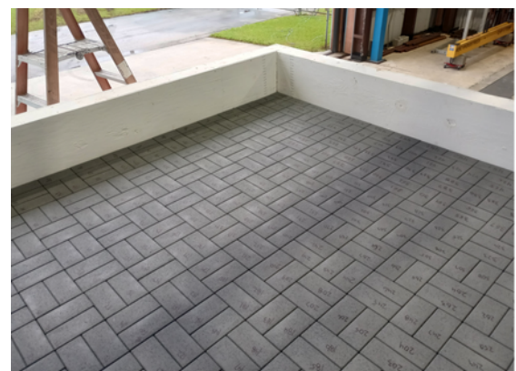
INSTALLED PAVER ASSEMBLY
